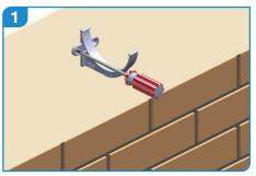
Identify the highest and lowest point of the gutter run and install brackets on each end ensuring a minimum fall of 1:600.
